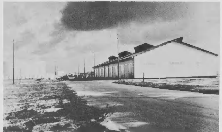
The first industrial building in the Oranjestad Free Zone was opened on October 31, 1972. The building will serve as an international distribution center to house storage, assembling and packaging operations directed mainly for export. Built by the Firm of Holman & van Eerden, the project costing Fls. 337,700 was financed by Holland under the 1st Phase of the Multi-Year Plan. The fenced-in area of the Free Zone is 6 acres, with some three acres adjacent to that area. E promer edificio industrial den Zona Libre di Oranjestad a ser habri Oct. 31. E edificio lo sirbi como un centro internacional di distribucion pa varios operacion di exporte. Traha pa Firma Holman & van Eerden, e proyecto a costa Fls. 337,700 y tabata financia pa Promer Fase di e Plan di Desaroyo di Multi-Anjas.
